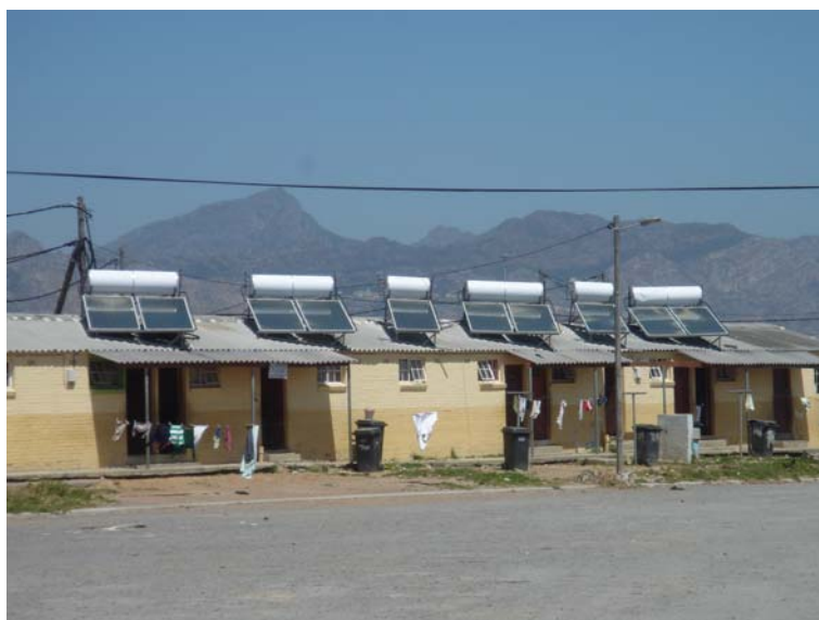
Solar water heaters in Lwandle – part of the “Hostel-to-Homes” renovation project.
